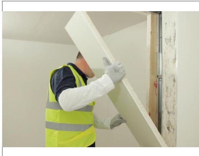
Figure 4 Window reveal installation
